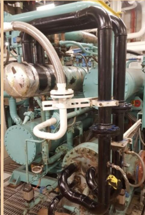
Here is an example of **refitting** of the **pipings insulation** of a refrigeration facility. In order to increase as maximum as possible the piping lifetime we provide a **turnkey service** that includes: chipping, first painting, second painting, insulation with armaxflex and then another painting over it to increase its resistance and lifetime.
