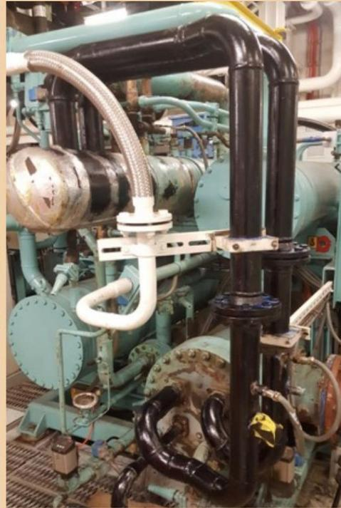
Here is an example of **refitting** of the **piping insulation** of a refrigeration facility. In order to increase as maximum as possible the piping lifetime we provide a **turnkey service** that includes: chipping, first painting, second painting, insulation with armaflex and then another painting over it to increase its resistance and lifetime.
